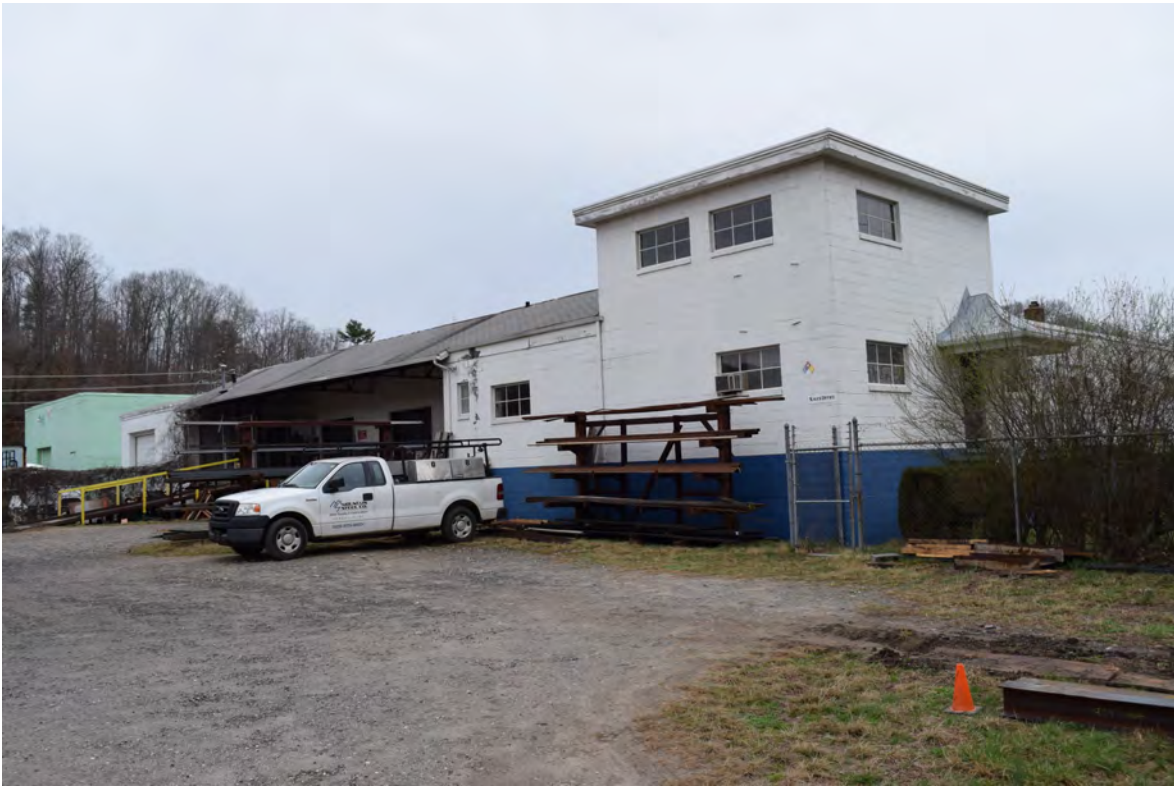
West elevation of W. R. Candler Transfer Company, view to the northeast
