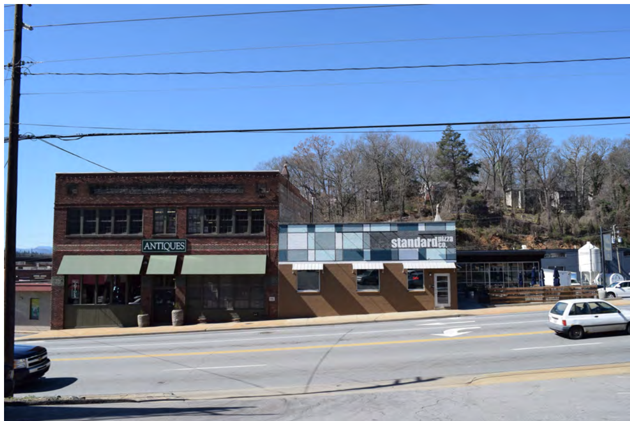
Blue Ridge Grocery, view to the west
