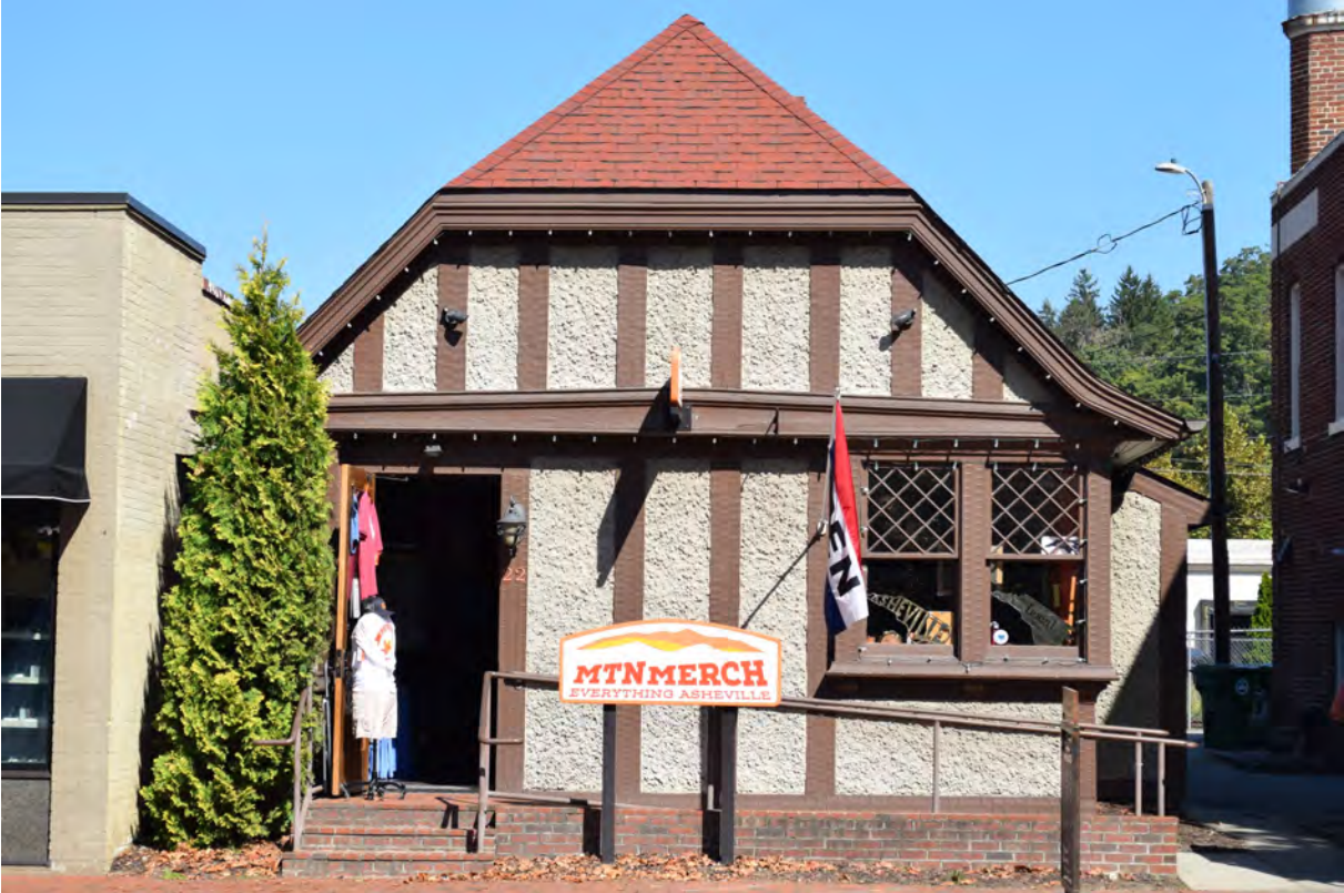
First Biltmore-Oteen Bank (NR 1979), 22 Lodge Street, view to the north
