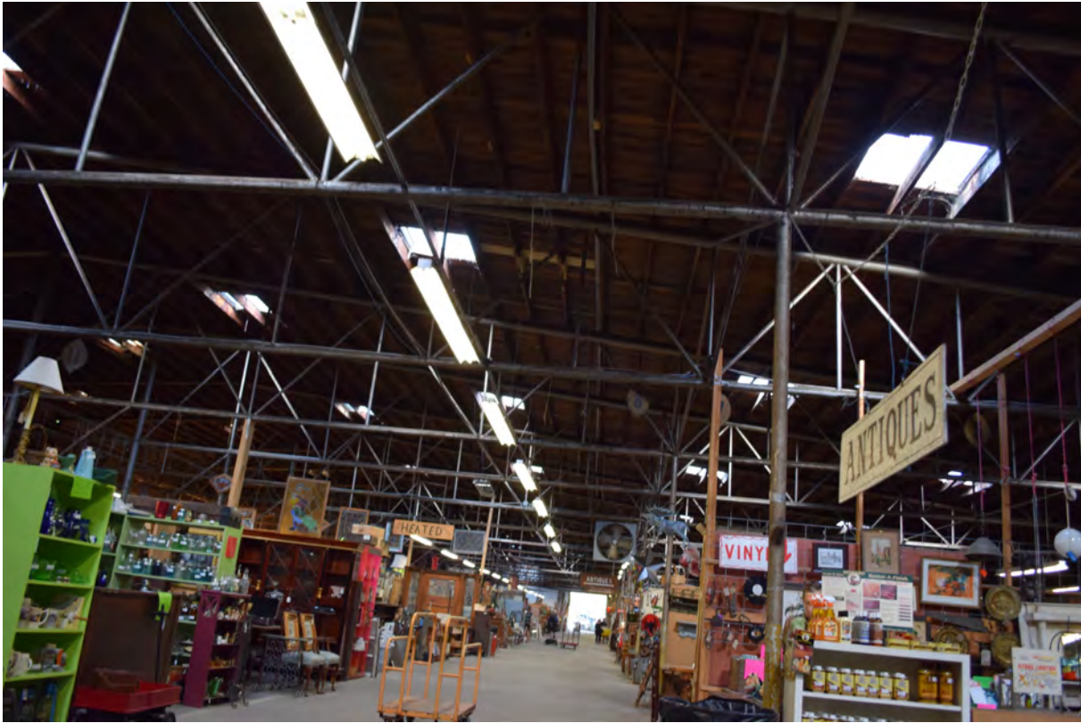
Interior of 1947 warehouse, view to the east
