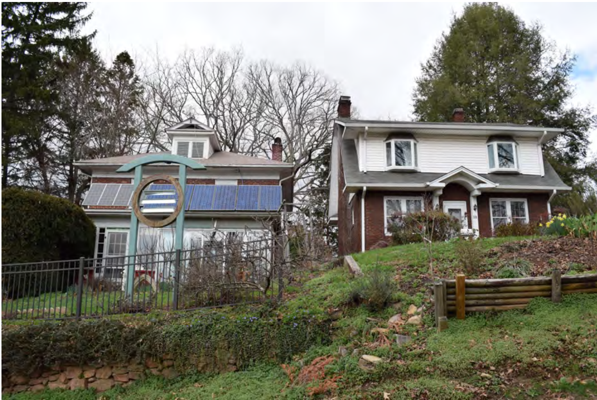
Arthur House (left) at 16 Finalee Avenue and C.C. West House at 18 Finalee Avenue, view to the north
