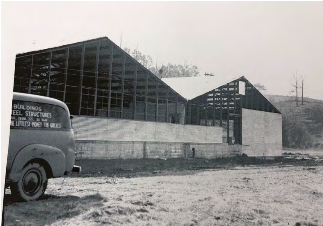
Buildings 1 and 2 under construction in 1953, south end, view to the northeast (from North Carolina Collection, Pack Memorial Library, Asheville)
