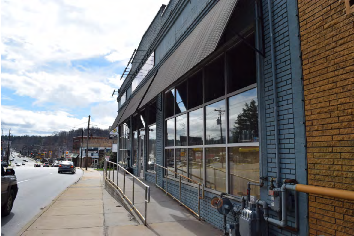
Facade looking south down Biltmore Avenue, view to the south-southwest
