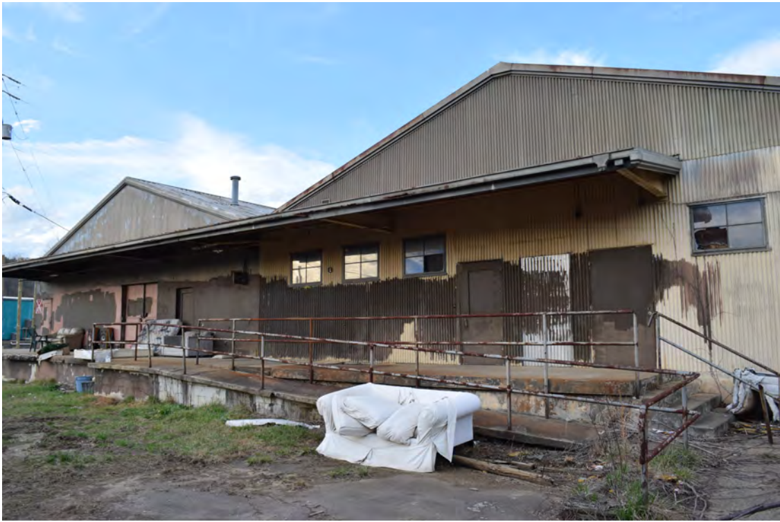
South end of buildings 1 and 2, view to the north-northwest
