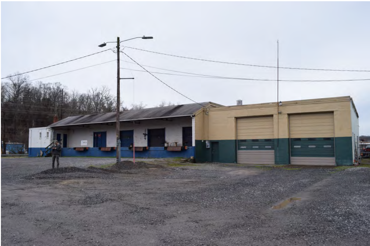
East elevation of W. R. Candler Transfer Company, view to the west-southwest
