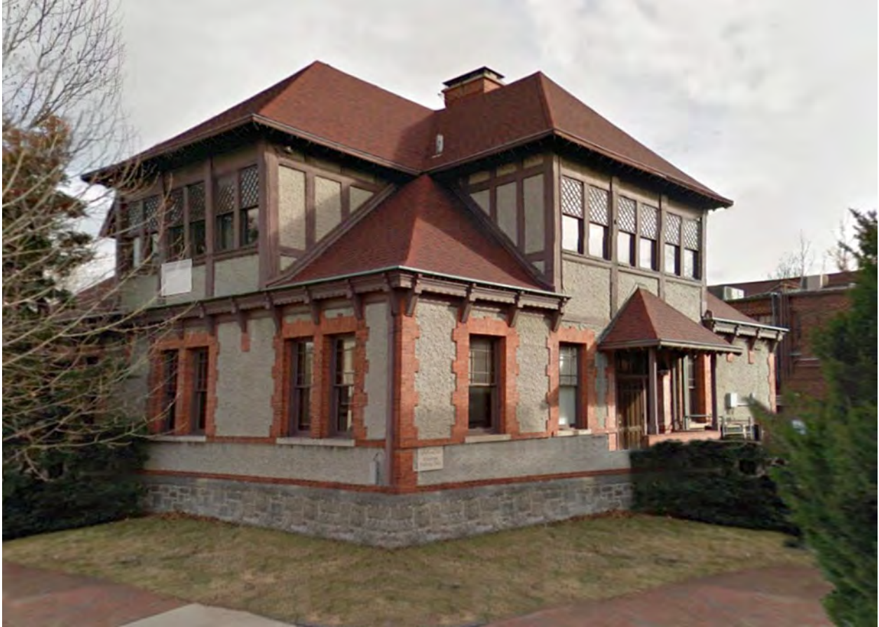
Northwest (rear) corner, view to the southeast
