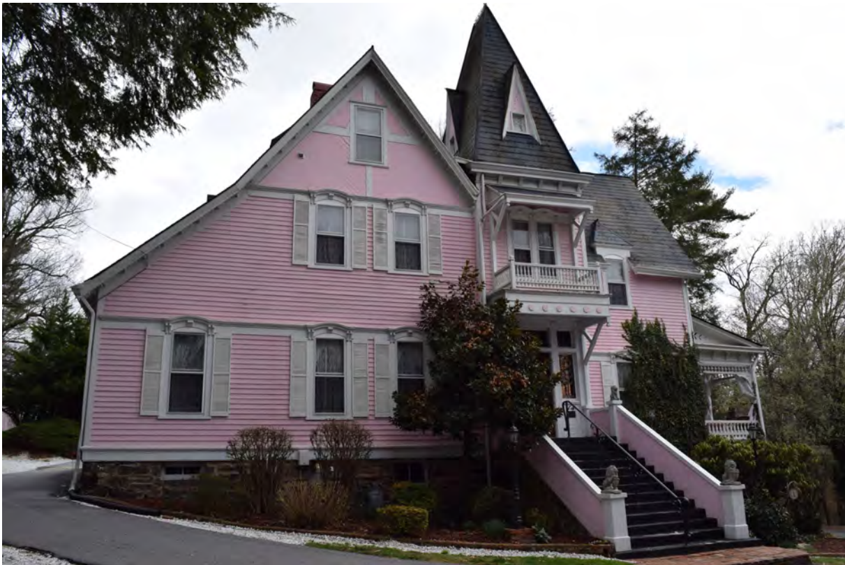
William E. Breese Sr. House facade, view to the east-southeast
