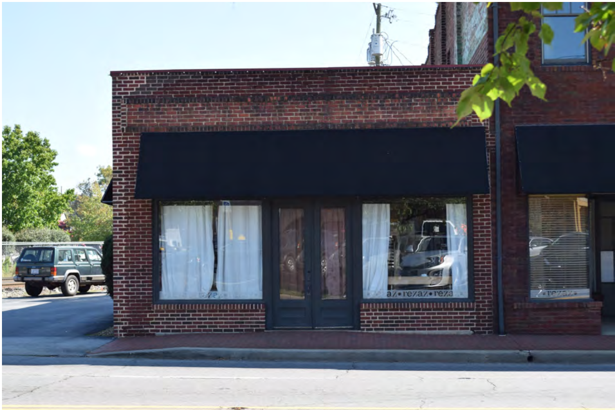
One-story wing built circa 1927, view to the east
