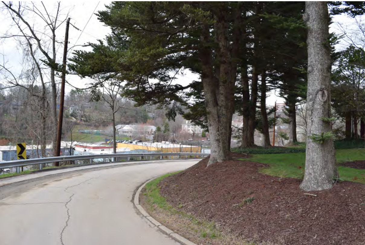
Finalee Avenue, view to the northwest toward Biltmore Avenue
