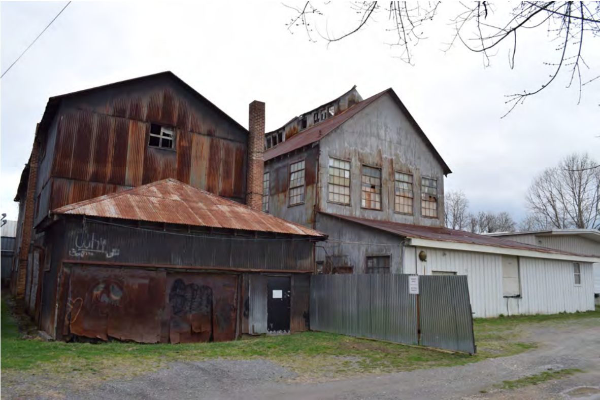
Two processing buildings south of main building, view to the southeast
