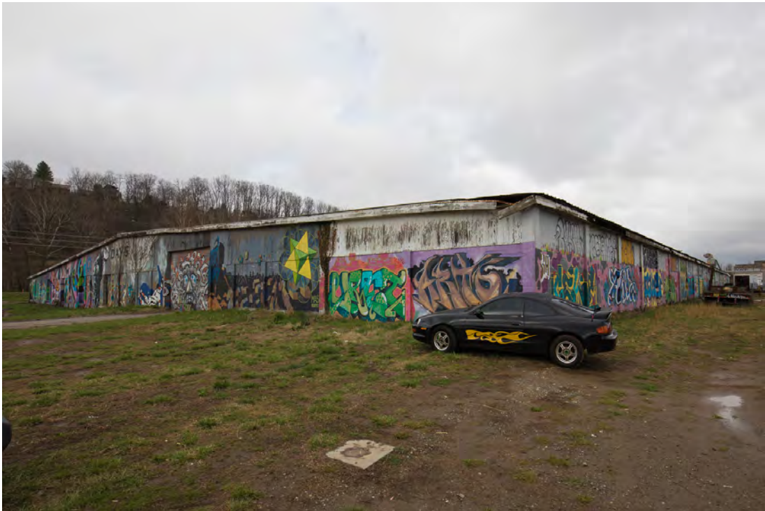
Big Burley Tobacco Warehouse (1953), view to the northwest
