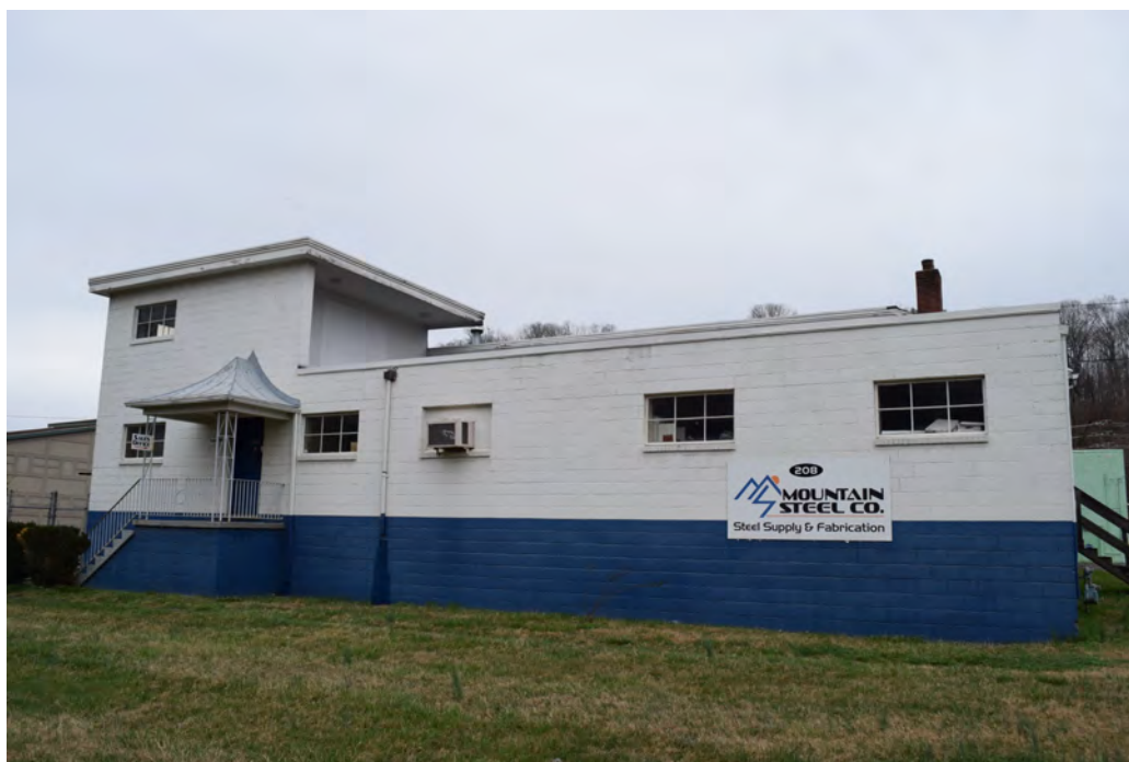
Façade (south elevation), view to the north-northwest
