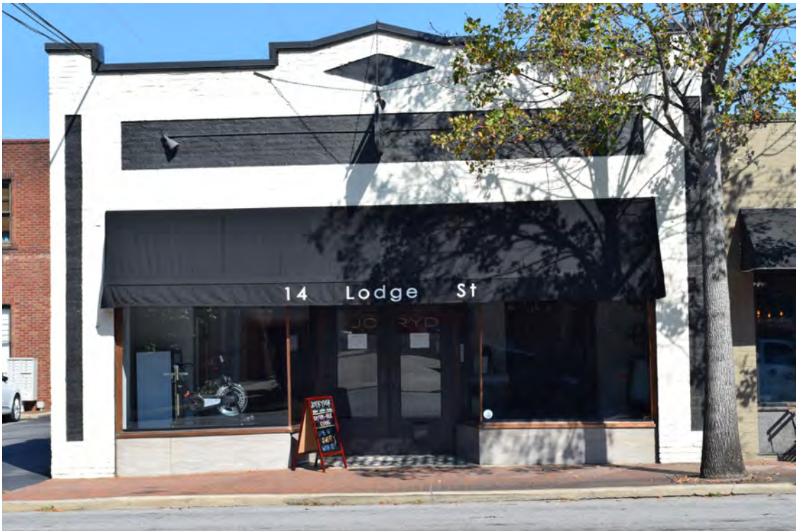
Commercial building (BN5550) at 14 Lodge Street, view to the north
