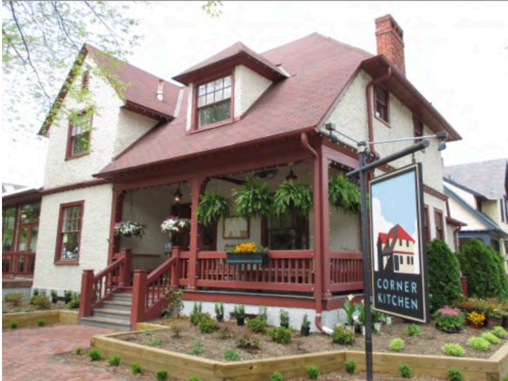
Cottage (BN0167, NR 1979) at 3 Boston Way, view to the northeast
