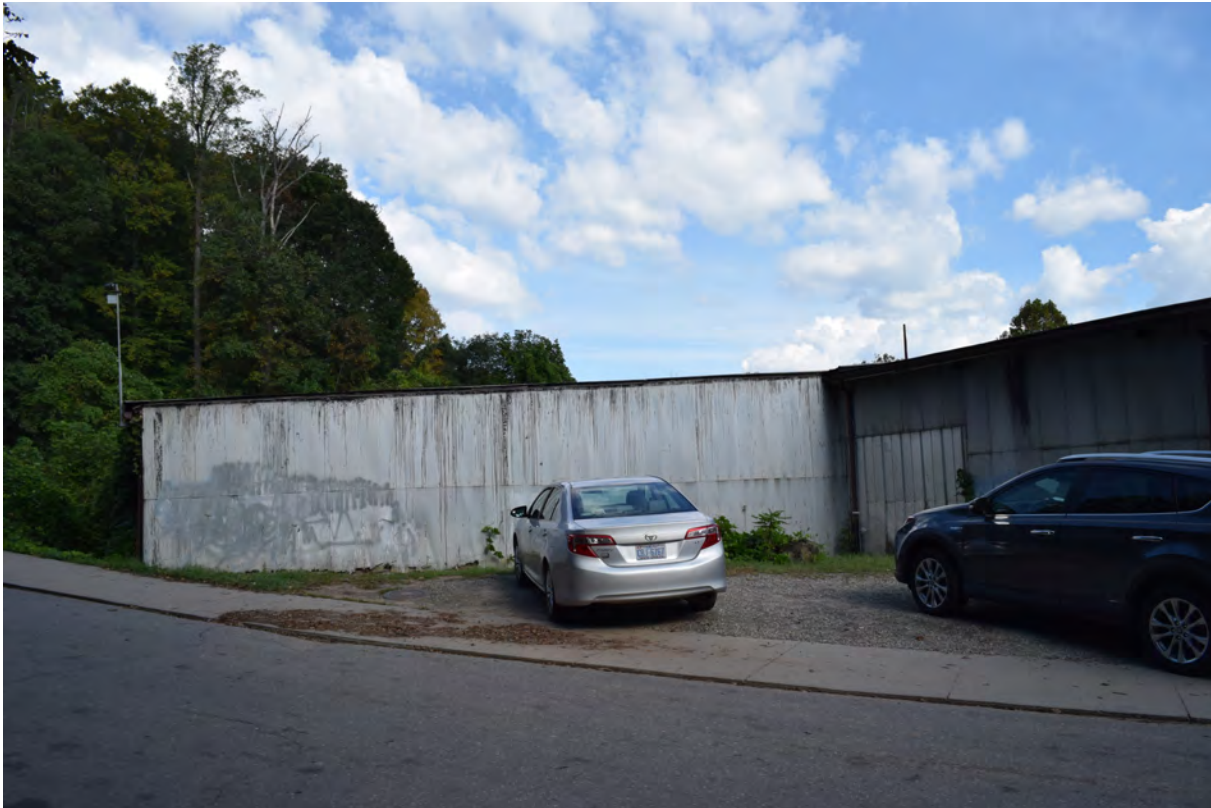
North elevation addition, view to the east
