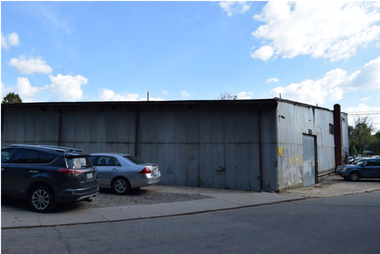
Northwest (front) corner, view to the south-southeast from Caledonia Road
