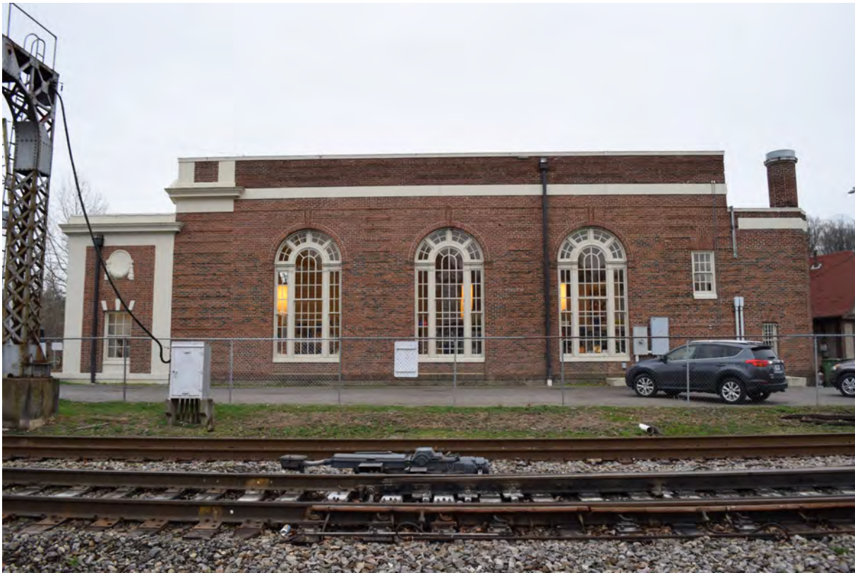
Biltmore-Oteen Bank, rear elevation, view to the south
