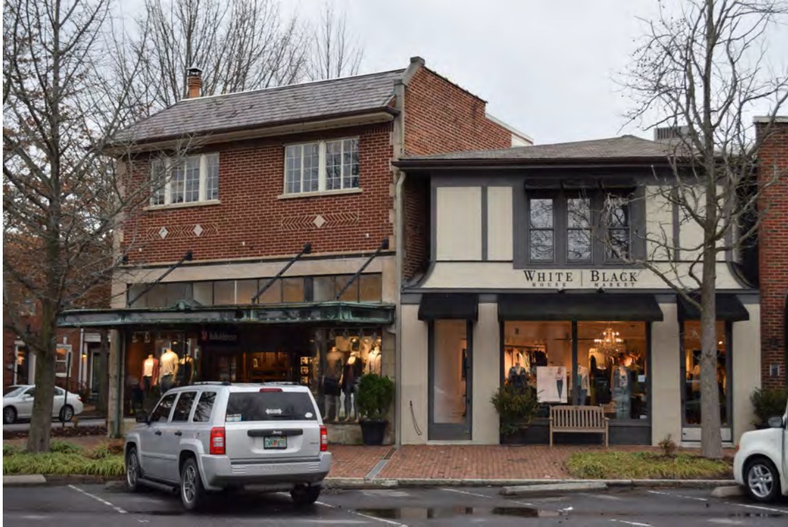
1 Kitchin Place (1926) and 3 Kitchin Place (1929), view to the southeast
