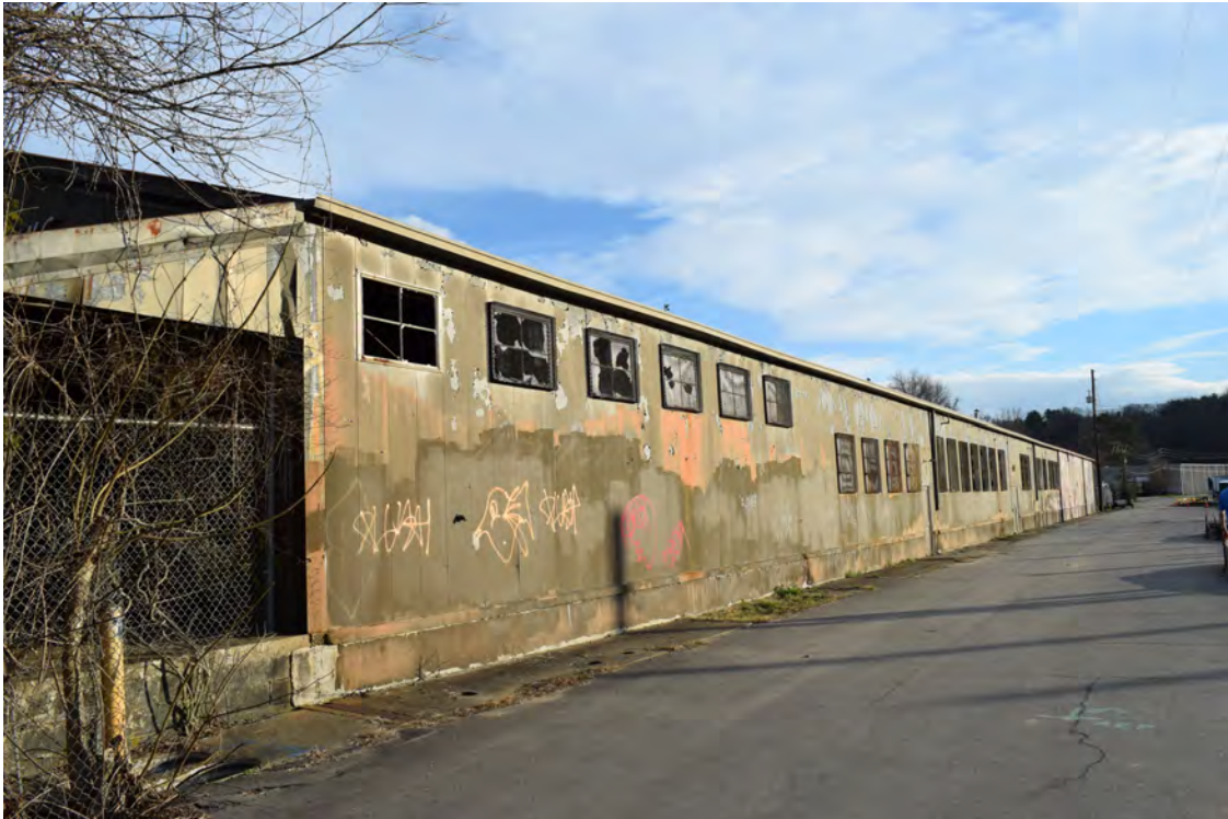
West elevation of building 1 along Simpson Street, view to the south-southeast
