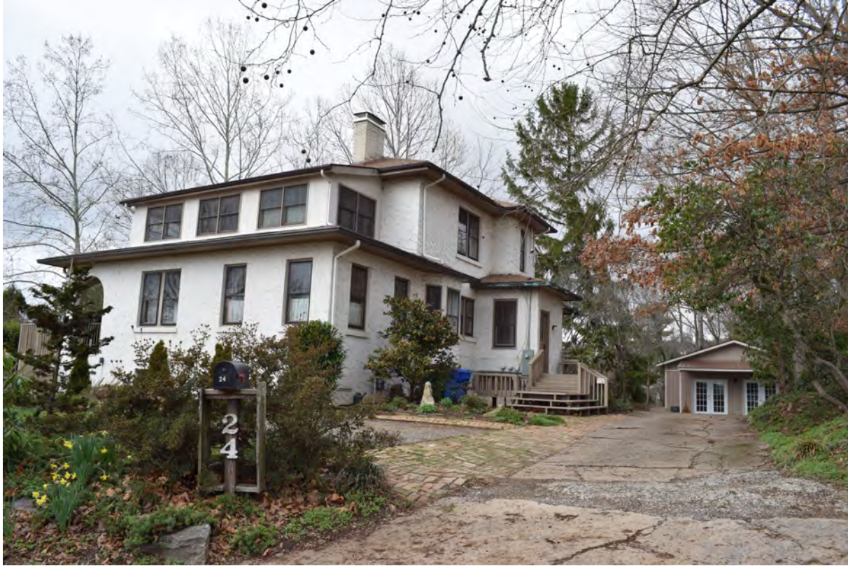
Reeves House at 24 Finalee Avenue, view to the northwest
