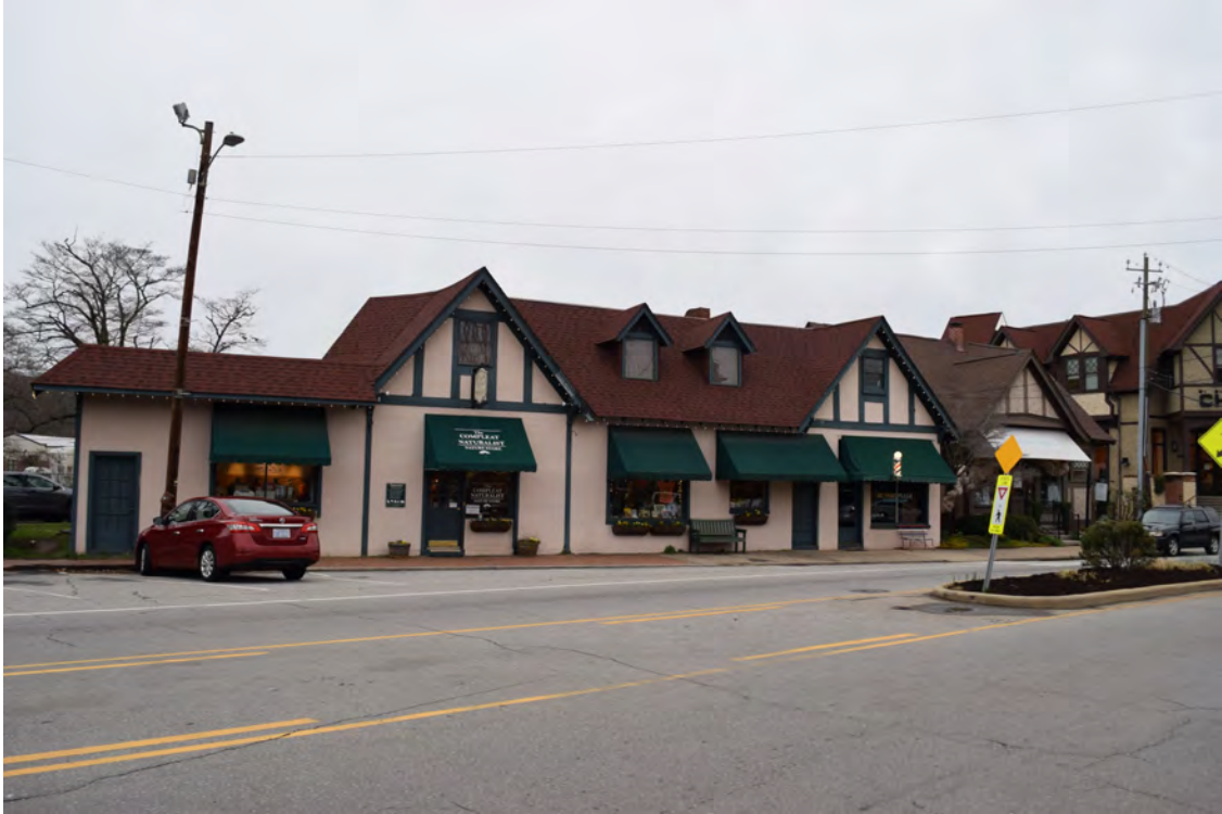
Biltmore Village Commercial Buildings (BN0153, NR 1979) at 2 Brook Street, view to the southeast
