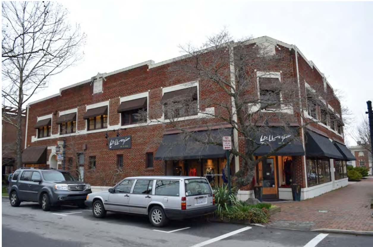
McGeachy Building, view to the northwest
