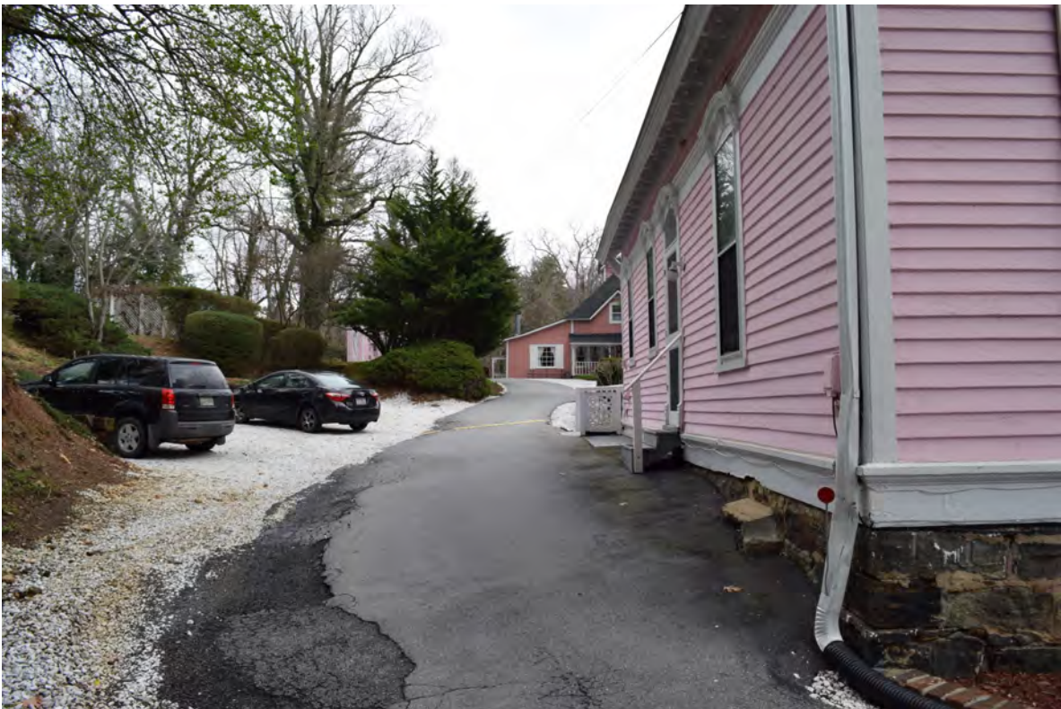
North side of the William E. Breese House, view to the east
