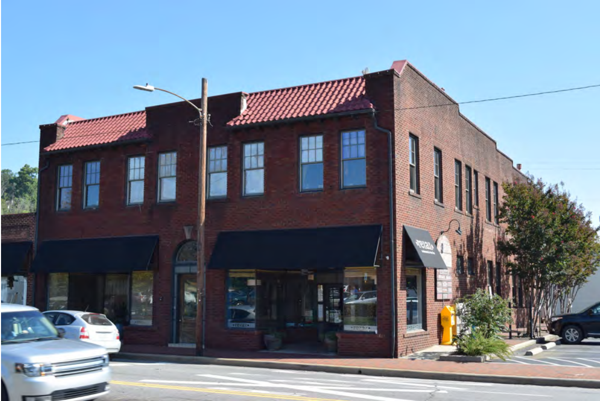
Biltmore Hardware Building (BN0928, NR 2003) at 28-32 Hendersonville Road, view to the northeast
