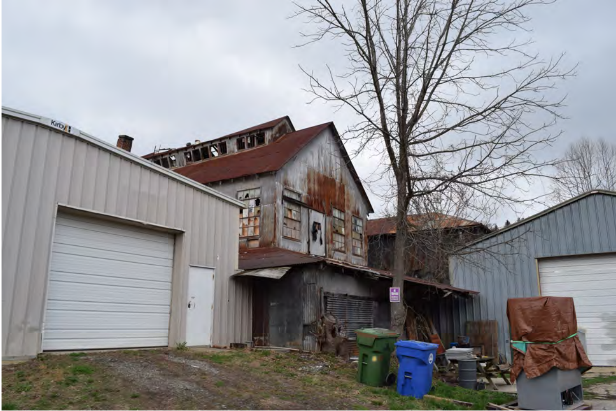
Two modern warehouses and rear corner of southernmost processing building, view to the northwest
