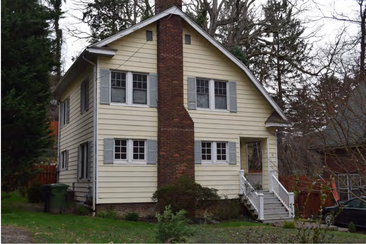
Crawford House at 3 Kenilwood Place, view to the southwest
