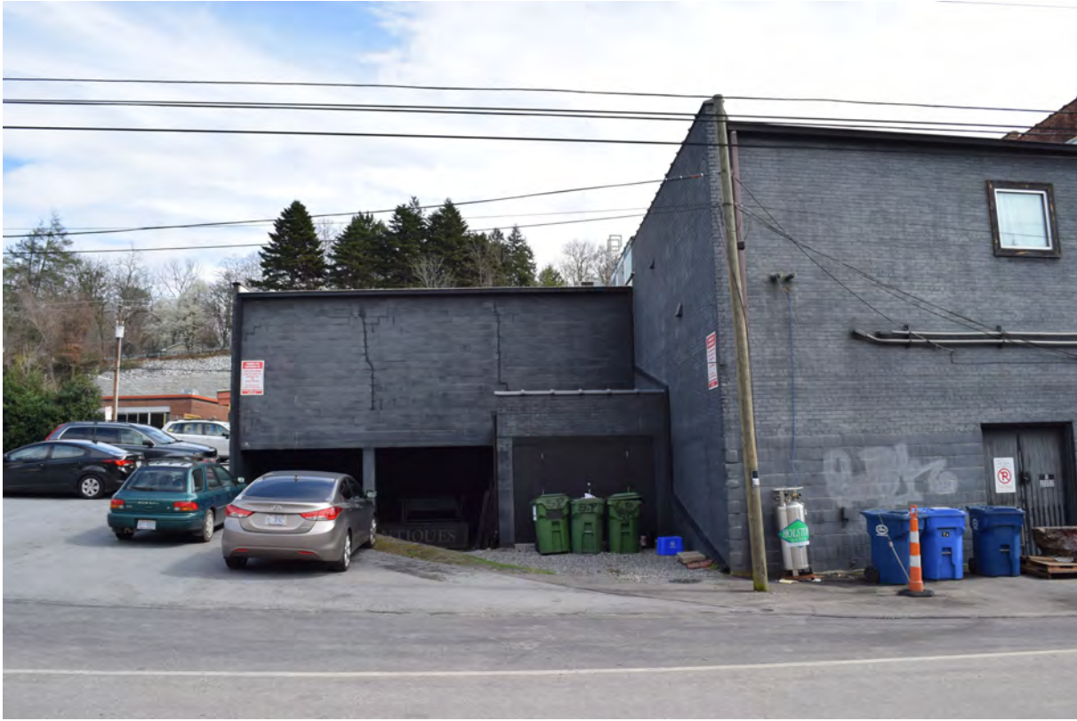
Rear of modern addition to 1953 warehouse addition, view to the east
