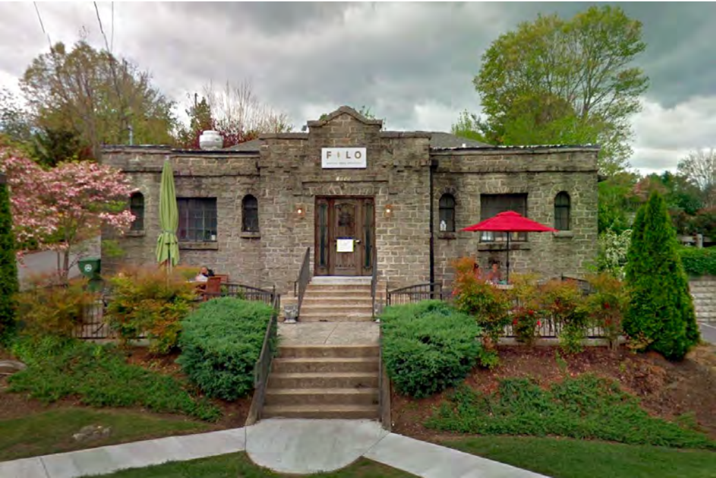
Former American Legion Post 70, 1155 Tunnel Road, Asheville, view to the south
