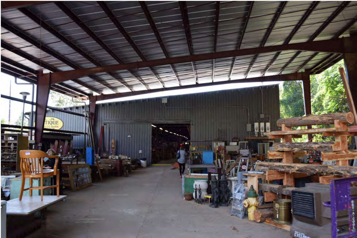
Open-sided shelter on the east elevation, view to the west
