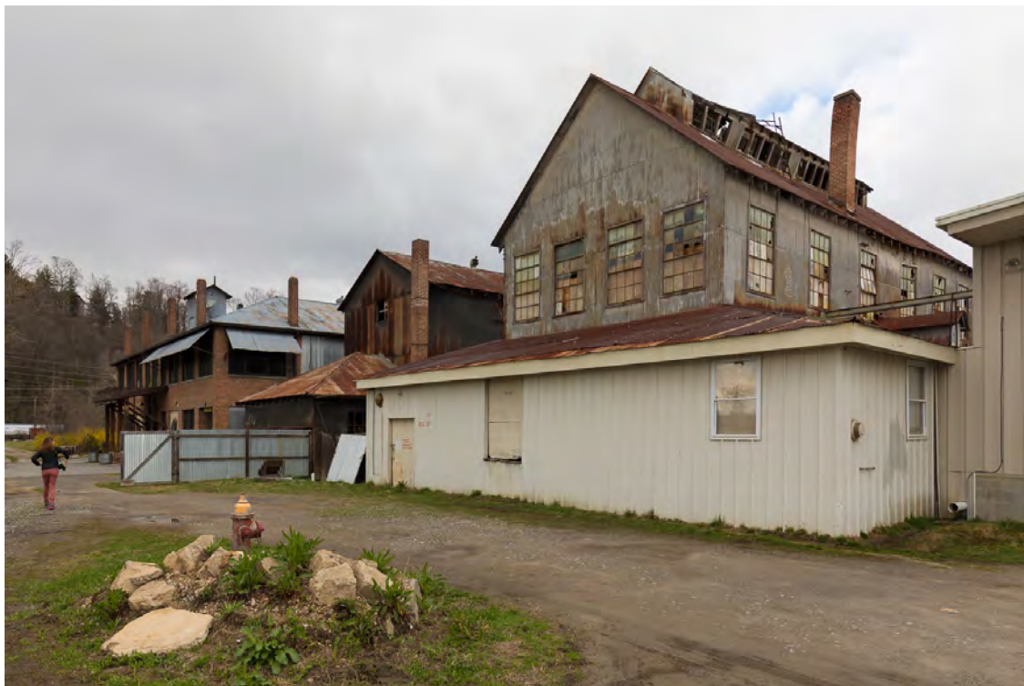
Asheville Mica Company buildings from 1916, view to the northeast
