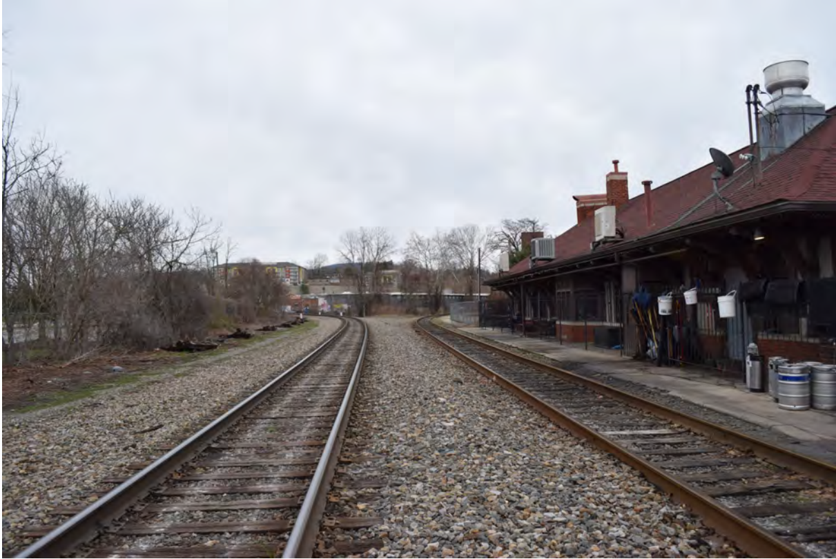
Tracks of the former Southern Railway with the depot to the right, view to the southeast
