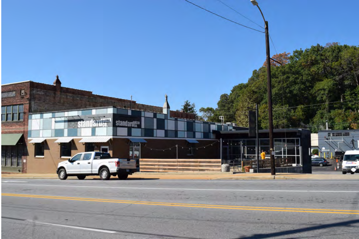
1953 addition to Blue Ridge Grocery, view to the west-southwest
