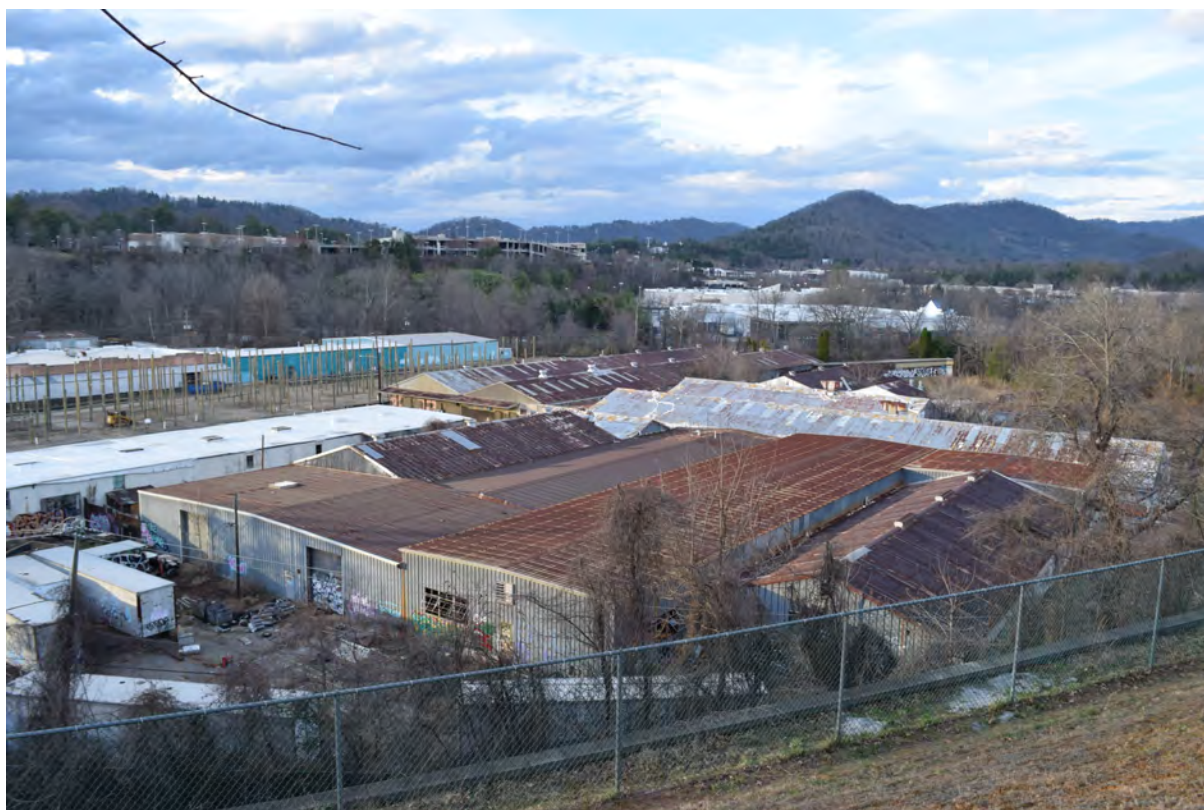
Overview of Three Mountaineers, view to the north
