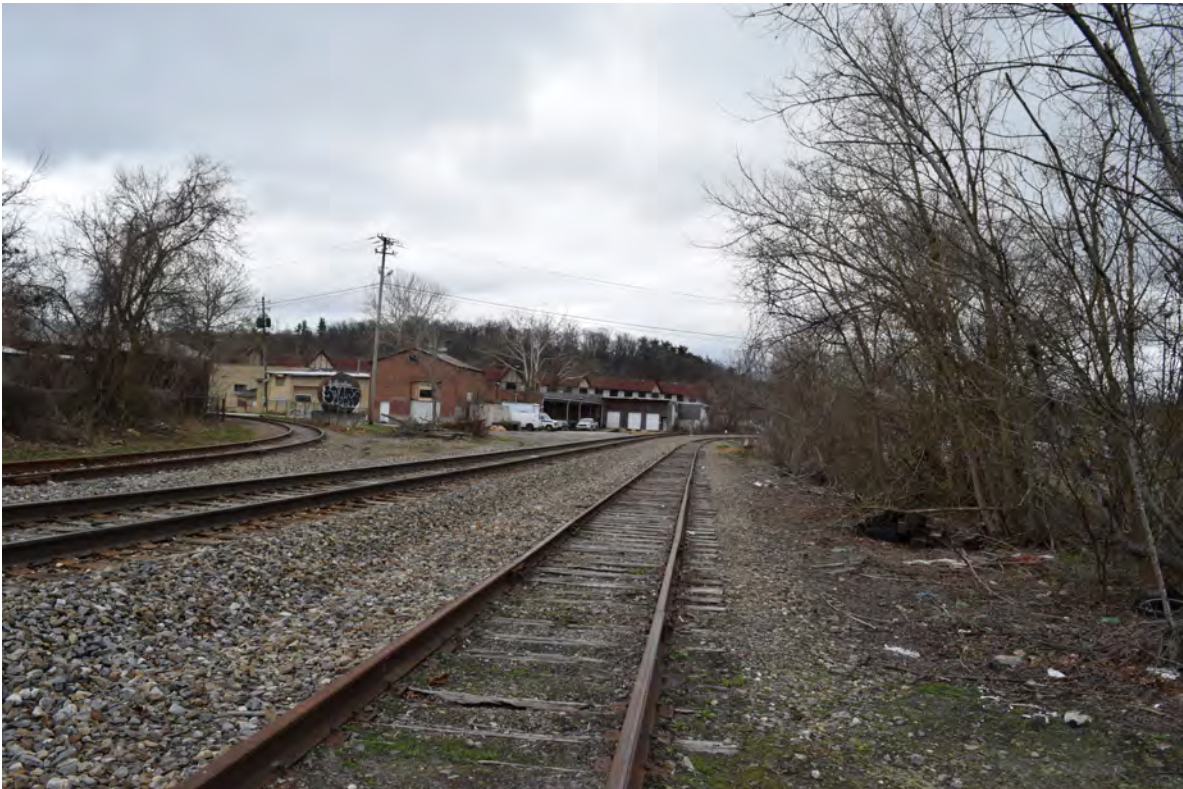
The tracks of the former Southern Railway extend along the south side of the project area, view to the west toward Biltmore Village
