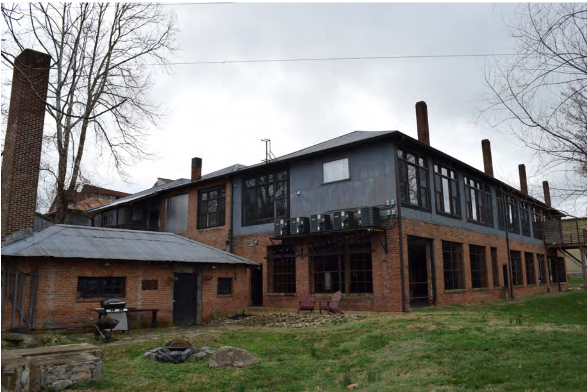
Smelter building and main building, view to the southwest
