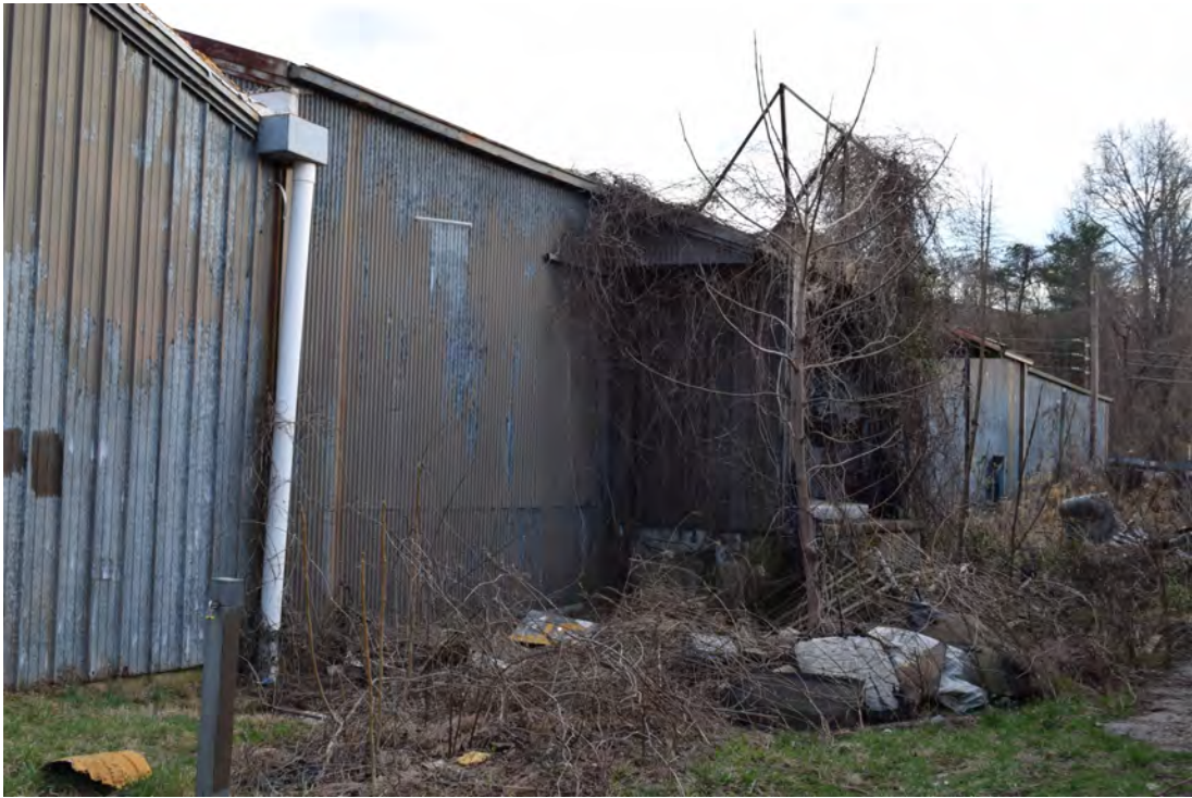
West elevation of building 6, view to the south
