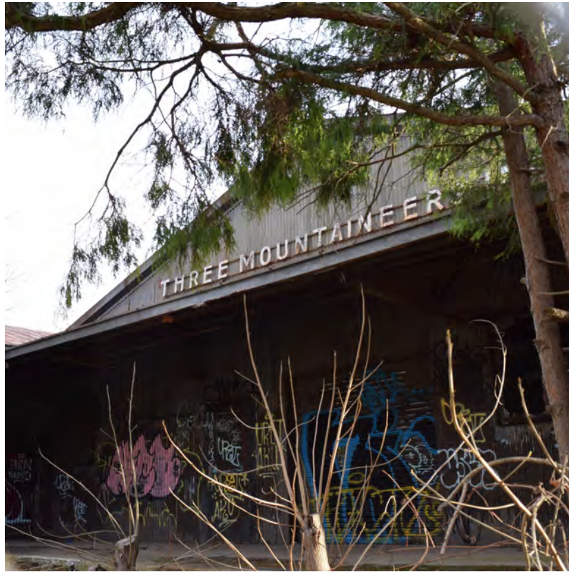
North end of the original building (building 1), view to the southeast
