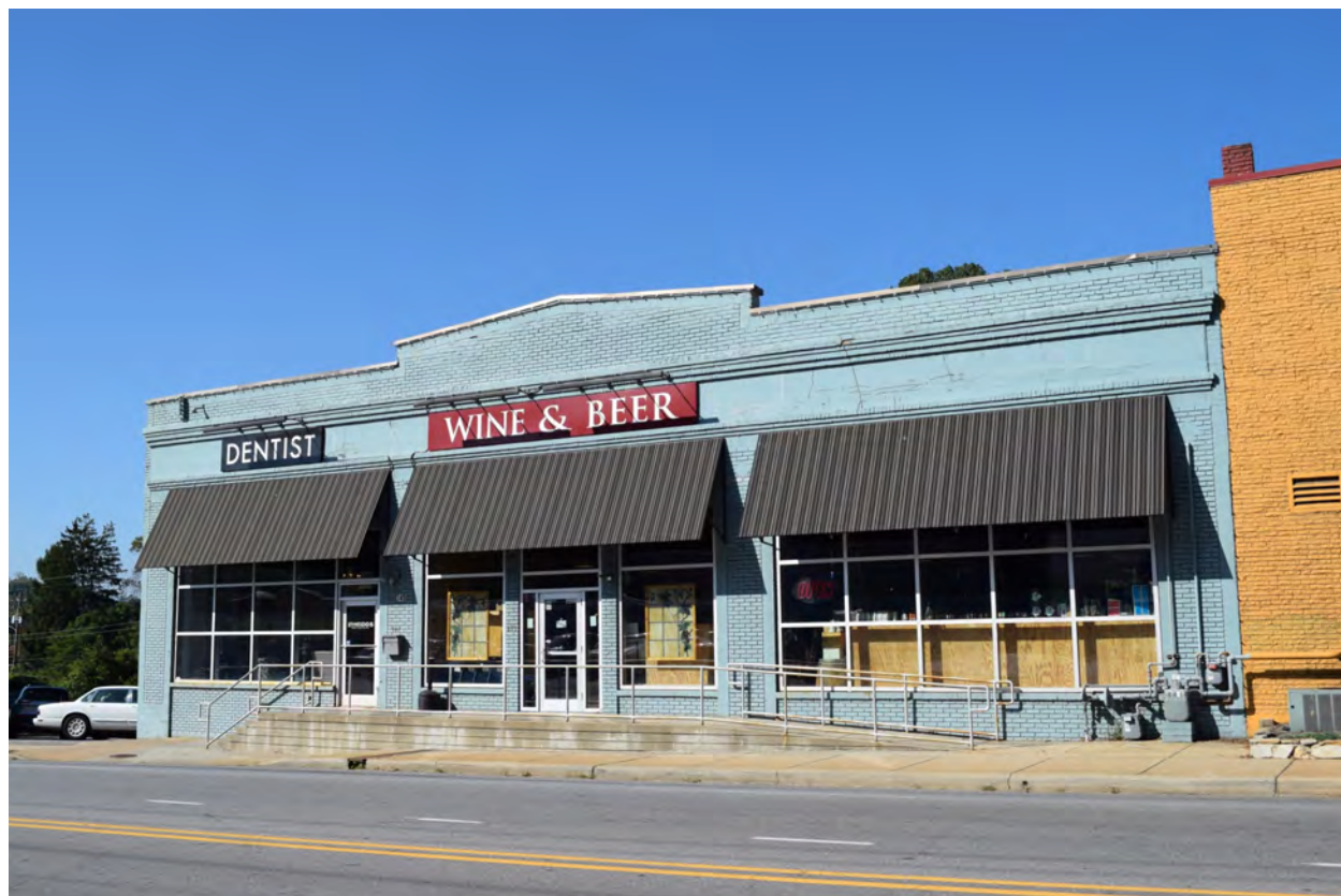
Southern Paper Products Company, view to the west-southwest
